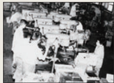
Factory at the time of establishment
